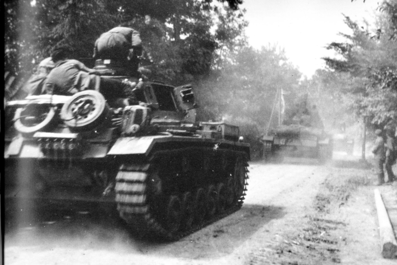
A column of heavily laden Pz.Kpfw.III's from the 46.Panzer-Korps during its furious drive on Belgrade in early April 1941. The crew have stowed a number of items over the engine deck, including supplies and rolled-up canvas sheeting. Note the spare wheels attached to the rear for additional armoured protection.
