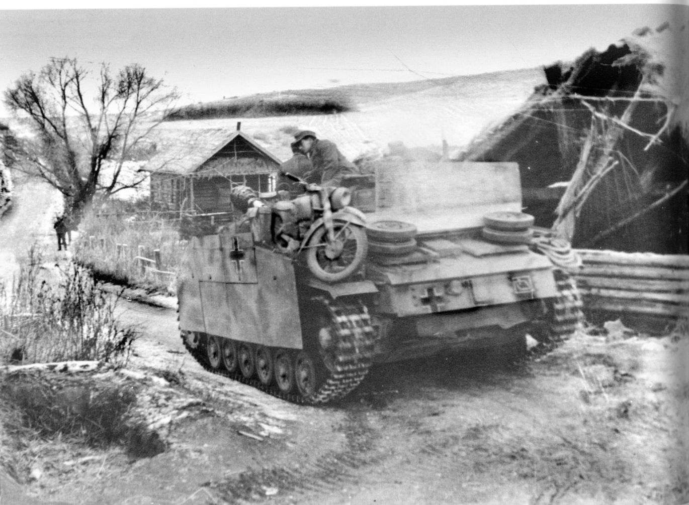
A StuG.III Ausf.G advances through a Belgian village during the later stages of the Ardennes offensive in January 1945. Note the BMW motorcycle attached to the StuG's offside rear. The stowage bins mounted on the engine deck can be seen left in an open position.
