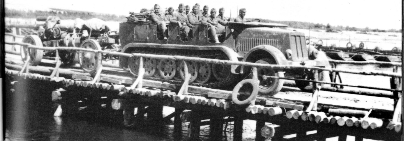
An Sd.Kfz.7 towing a 15cm sFH heavy field howitzer passes over a river on a wooden bridge built by German pioneers to carry heavier armour. Note the pontoon bridge erected alongside the wooden bridge. This was built in order carry lighter loads in the Panzer divisions.
