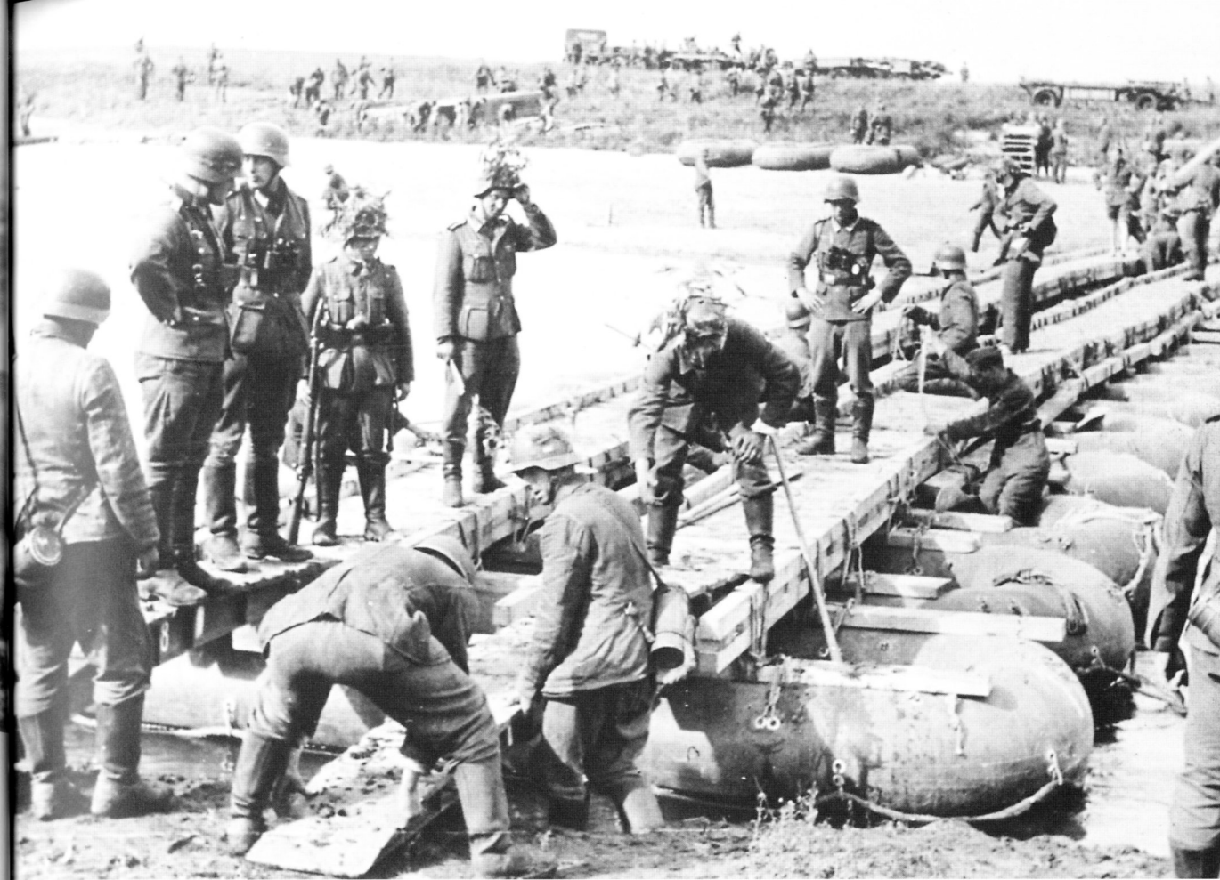
Engineers prepare for the crossing of support vehicles on a hastily erected pontoon bridge. This bridge has been lashed together with inflatable boats. For river crossings under fire, inflatable boats were used for assault, and then relegated to bridging or ferrying.
