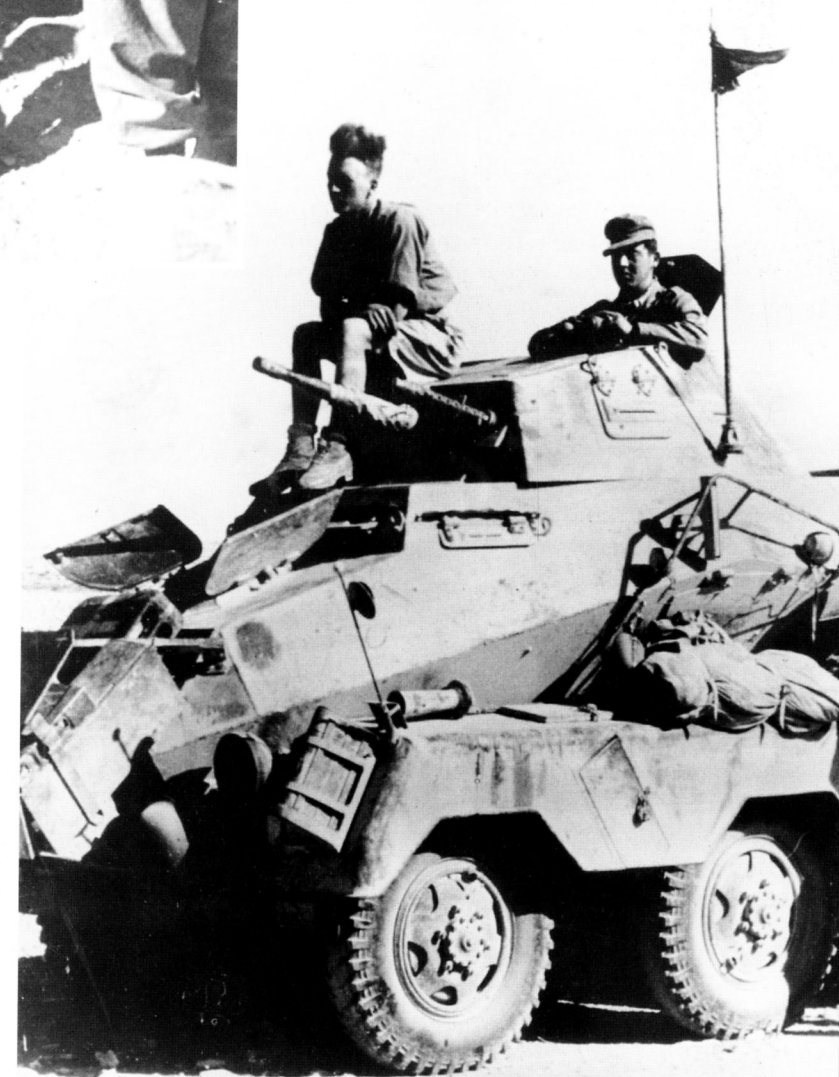
An eight-wheeled Sd.Kfz.231 heavy armoured car during operations in July 1941. These vehicles were unique among German armoured cars in the Panzer divisions. All eight wheels were individually powered, which ensured that the vehicle could still move even after enemy fire damaged one or more of its wheels.
